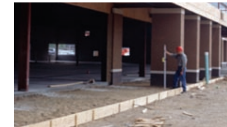
Forms and Footings
